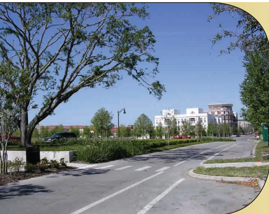
The curb extension to this New Broad Street crosswalk in Baldwin Park, Florida, shortens the crossing distance for pedestrians.
