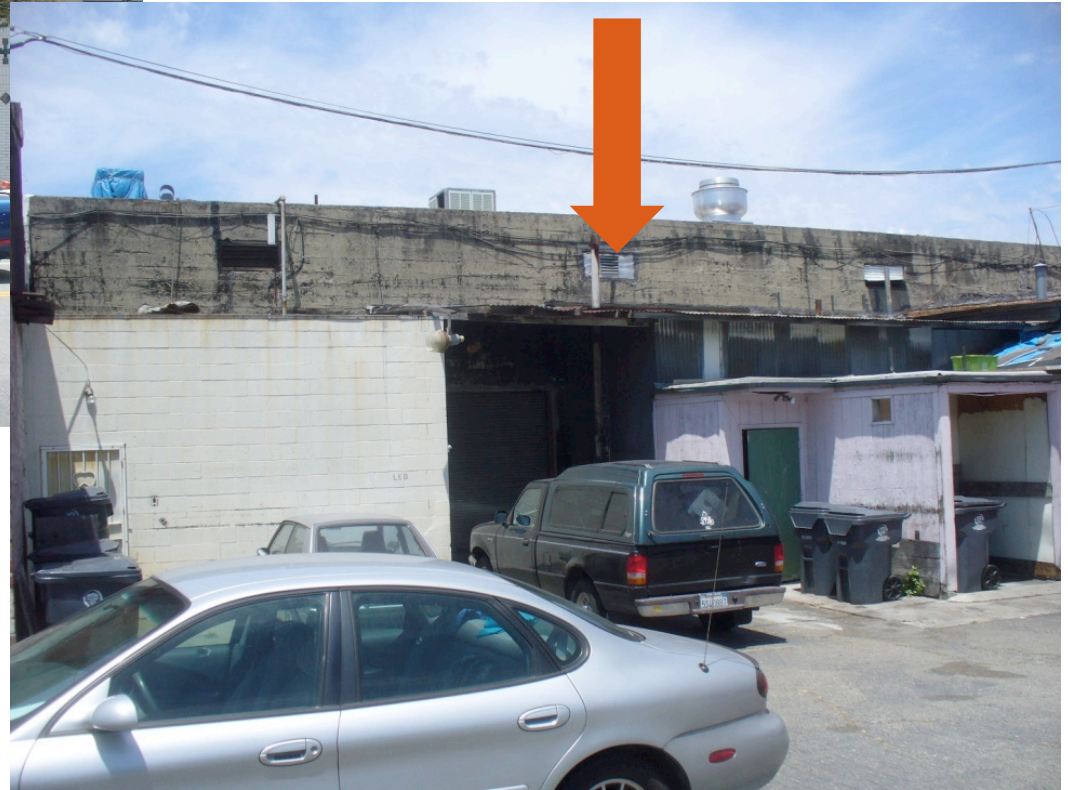
Concrete in the back
